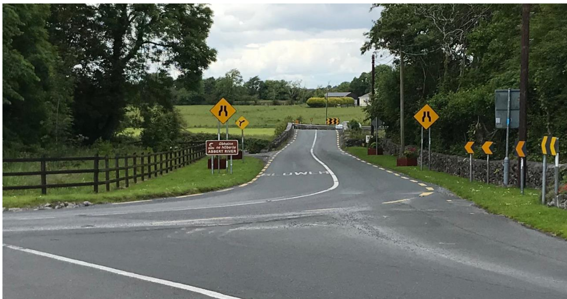
Figure 2-4 N63 Eastbound approaching Liss Bridge
