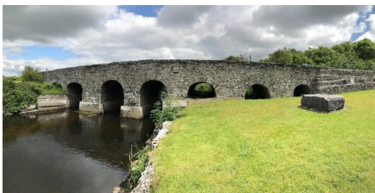
Figure 2-1 Existing N63 Liss Bridge with patchwork parapet repairs.
